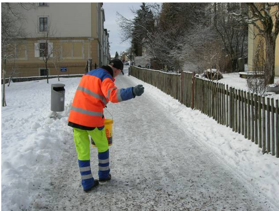
Photo 3 - Hand spreading
